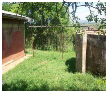
Figure 6: Cement tank in Tulimani division
