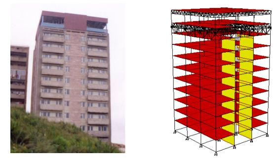
**Figure 1.** General view of the apartment building, the seismic resistance of which has been increased by the method of additional seismic isolated upper floor (proposed by the author of this paper), and the design model of
